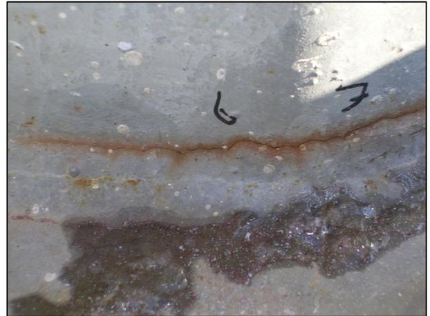
**Toe Cracks at Upper Toe of Weld in Pole Shaft at Polygonal Bend Line (Visible Rust)**
