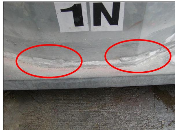
**Manufacturer Repair or Reinforcement of Upper Toe of Base Weld Observed in Field**
