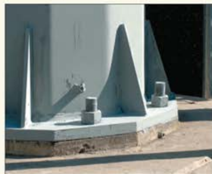
Base plate with stiffeners.
