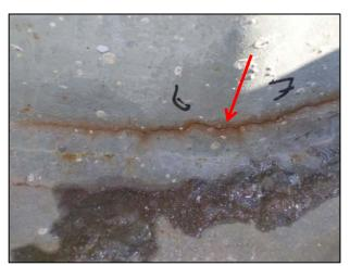
Toe Cracks at Upper Toe of Weld in Pole Shaft at Bend Line (Visible Rust)
