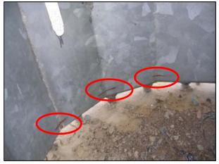
Socket Style Base Connection Toe Cracking Viewed From the Inside of the Pole (Visible Rust)
