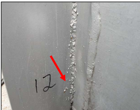
Weld Spatter at a Modification Stiffener and Field-Welded Port Installation
