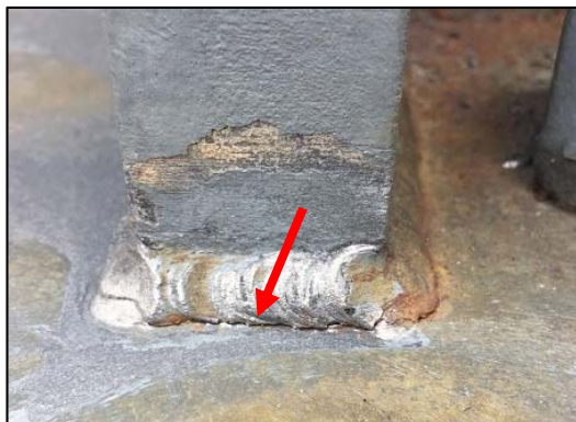
Base Plate Stiffener Weld Lower Toe Crack
