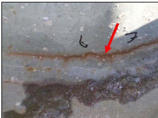
Monopole Base Plate Weld Upper Toe Crack
