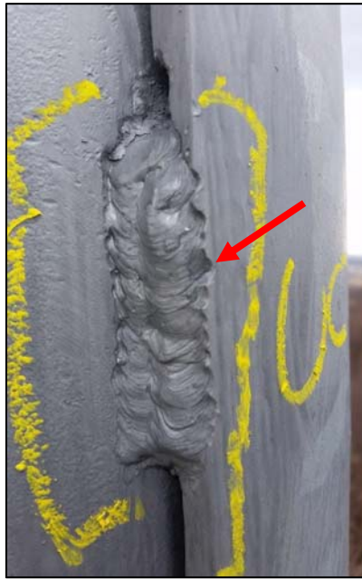
Tower Leg Split Pipe Stitch Weld Undercut
