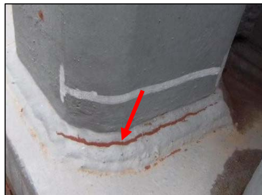
Anchor Rod Bracket Longitudinal Crack (Shown in Red)
