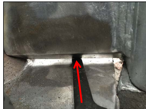
Root Gap to Base Plate Below Anchor Rod Bracket
