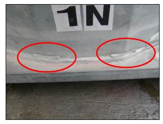
Manufacturer Repair or Reinforcement of Upper Toe of Base Weld Observed in Field
