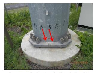
Manufacturer Toe Crack Repairs Visible in the Field
