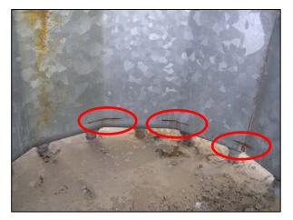
Socket Style Pole Base Through-Wall Toe Cracking Viewed From the Inside of the Pole (Visible Rust)
