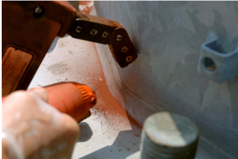
Magnetic Particle Test (MT) Powder at Revealing Toe Crack
